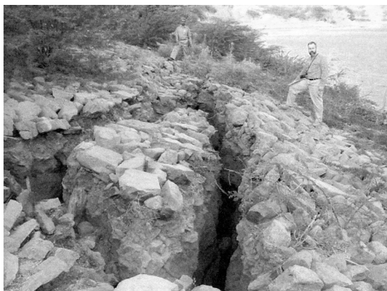
Fig. 11.3 Failure on upstream face of earthen dam
