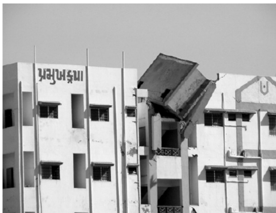
Fig. 11.8 Failure of water tank over the top of a multistorey building (Photo by Jaswant N. Arlekar)
