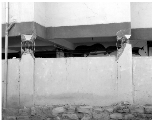
Fig. 11.7 Poorly compacted concrete due to congestion of reinforcement at the top of columns
