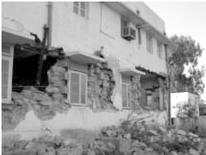
Fig. 11.4 Failure of a typical stone masonry building
